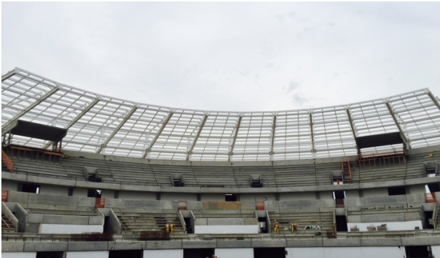
Fig. 9: Metallic beam fixed to the head of the columns.
