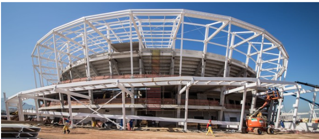
Fig. 10: External view of the Olympic Tennis Centre arena.
