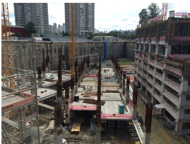
Figure 9. First phase of the precast columns installation.
